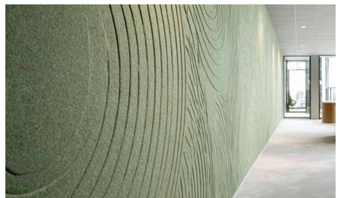
V-groove milling mounted on the wall
